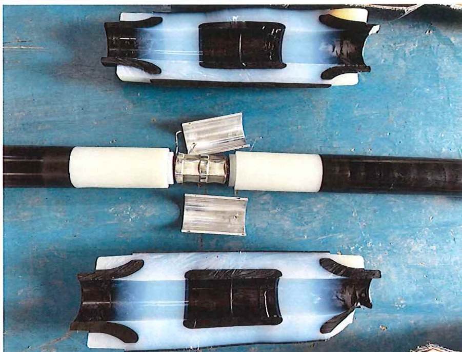
D7 直通接头检查 Examination for straight joint (1/2)
